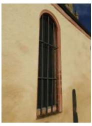
The one-piece semi-circular stone <u>window heads</u> on the south wall have been raised from their 1634 original position. This is indicated by the glazing check in the arch stones matching those in the lower window ingos.
